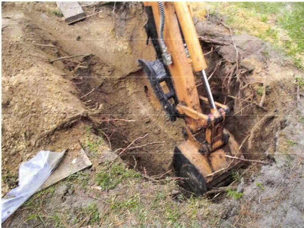
Picture 2: UST 1295Eagle removal in progress.
